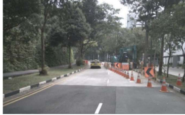
The decision is to maintain current speed and go straight is likely due to the presence of construction cones and a digger ahead, indicating ongoing road work that may require careful navigation and adherence to the current lane. The navigation command 'turn left' might be for a later point, as the immediate environment suggests caution rather than an immediate turn.
